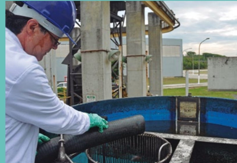
Left: waste in the grease traps at the Cedae treatment plant (Estação de Alegria). Above: biodiesel a product of the grease traps at the treatment plant
